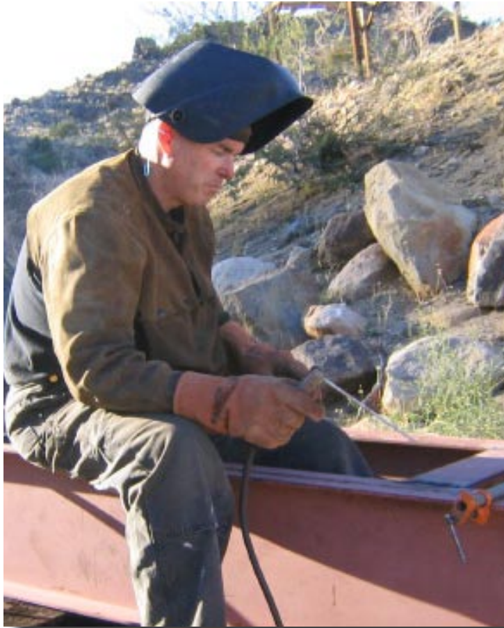
Roger Stabler welding on the 15" gauge bridge.
