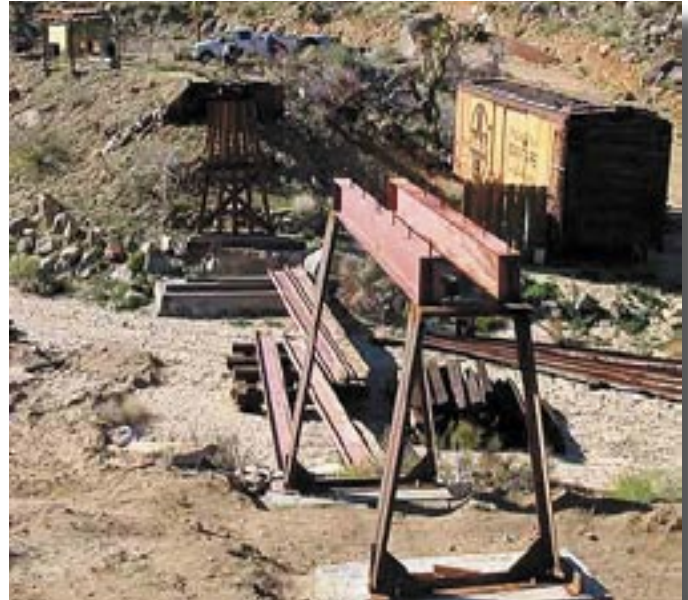
First span of Bridge #1 erected by Rick Mugele!
