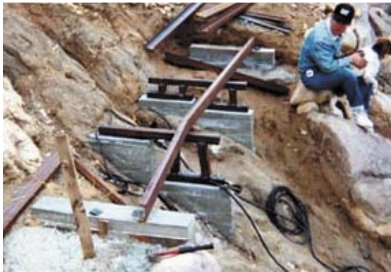
Greg Ratliff takes a break during bridge construction.
