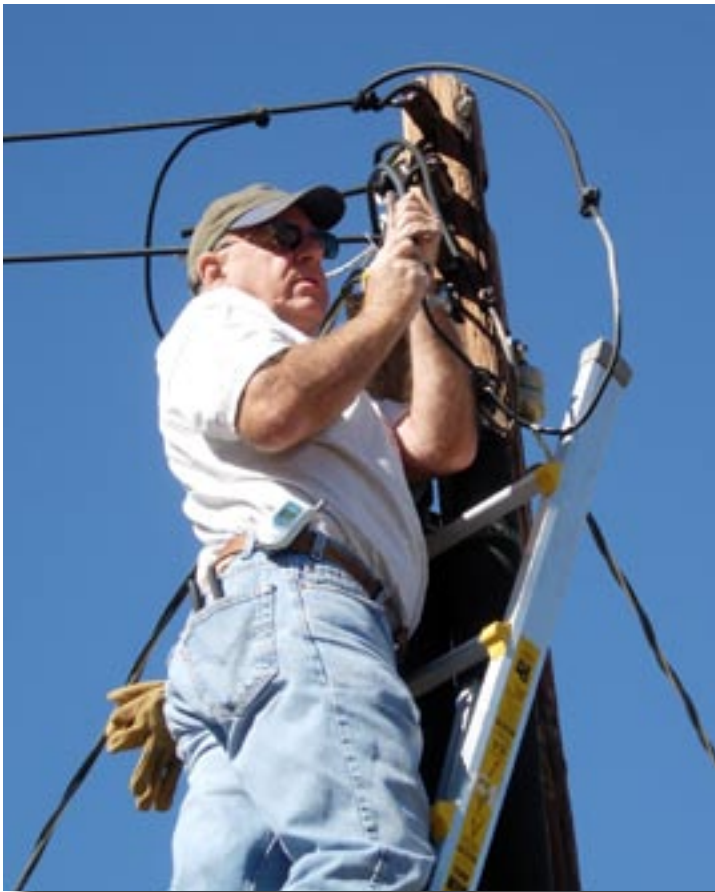
Tom Arnold cuts in the new power line to the Standard Gauge Cars. The old pole line up the hill was then removed.
