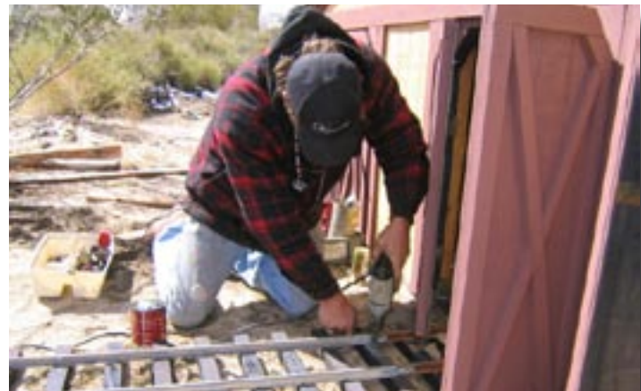
Paul Lavacot screws down the Car barn lead track.
