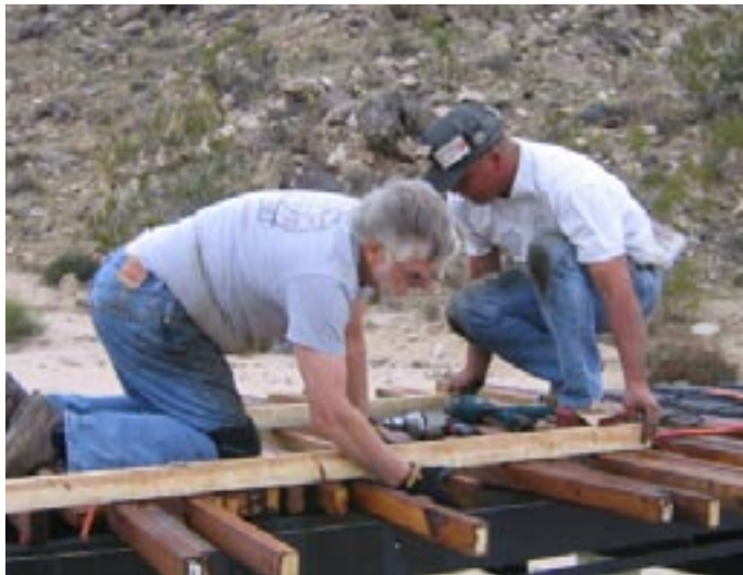
Peter Moseley and Brian Ratliff decking the Wye Bridge.
