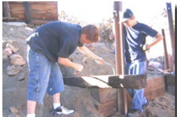
Joshua and Joseph Brehm cut timbers for the abutment wall.
