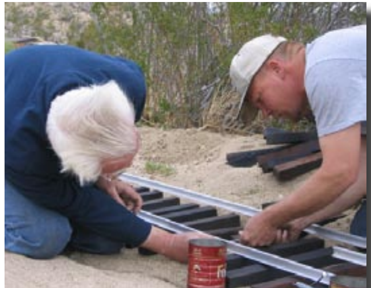
Ray Bjerrum & Greg Ratliff lay track for the new wye.
