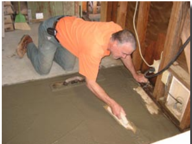
Bill Shepherd finishes the concrete floor in the Tedder Shed.
