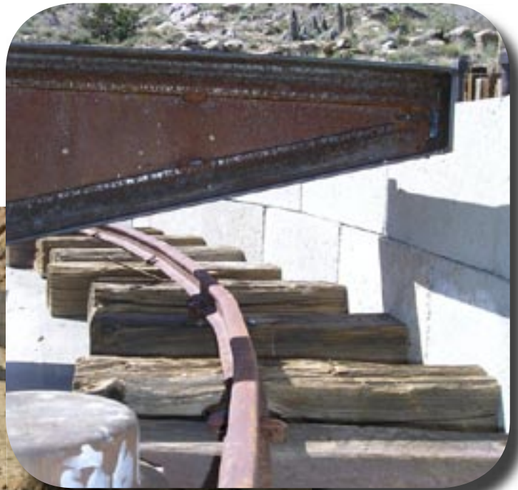
Ring rail is finally placed under the turntable bridge.
