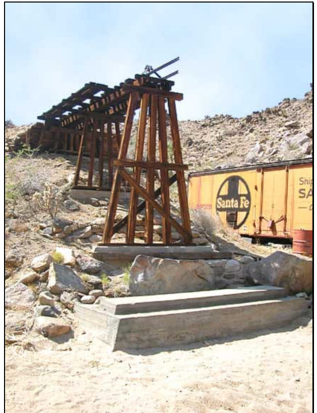
The completed West Pier on the GSD Bridge.
