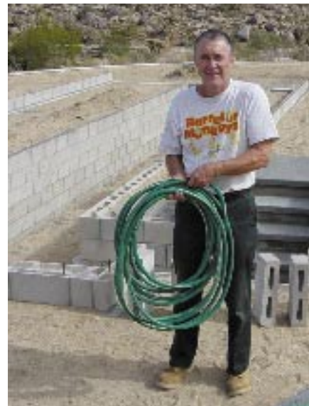
Bill Sheperd at the new Car barn foundation.
