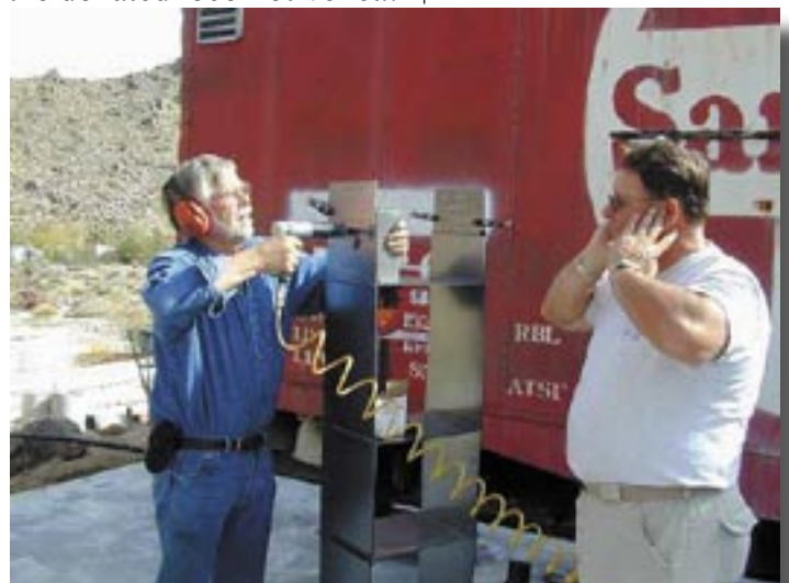
Peter and Ken riveting on the turntable bridge.
