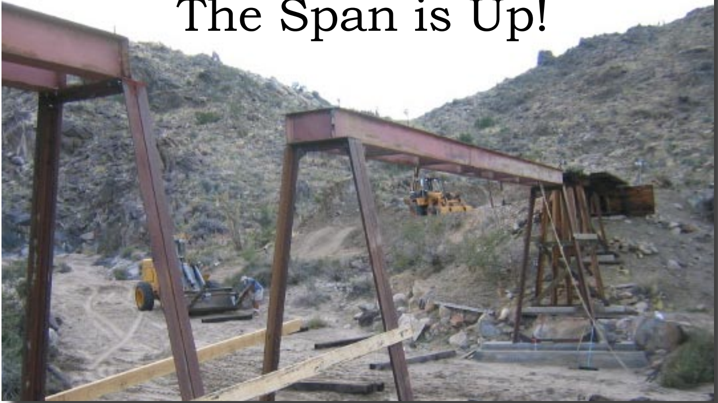
The 40' main span is up - thanks to Ole's loader!
